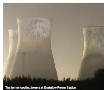
The former cooling towers at Drakelow Power Station
